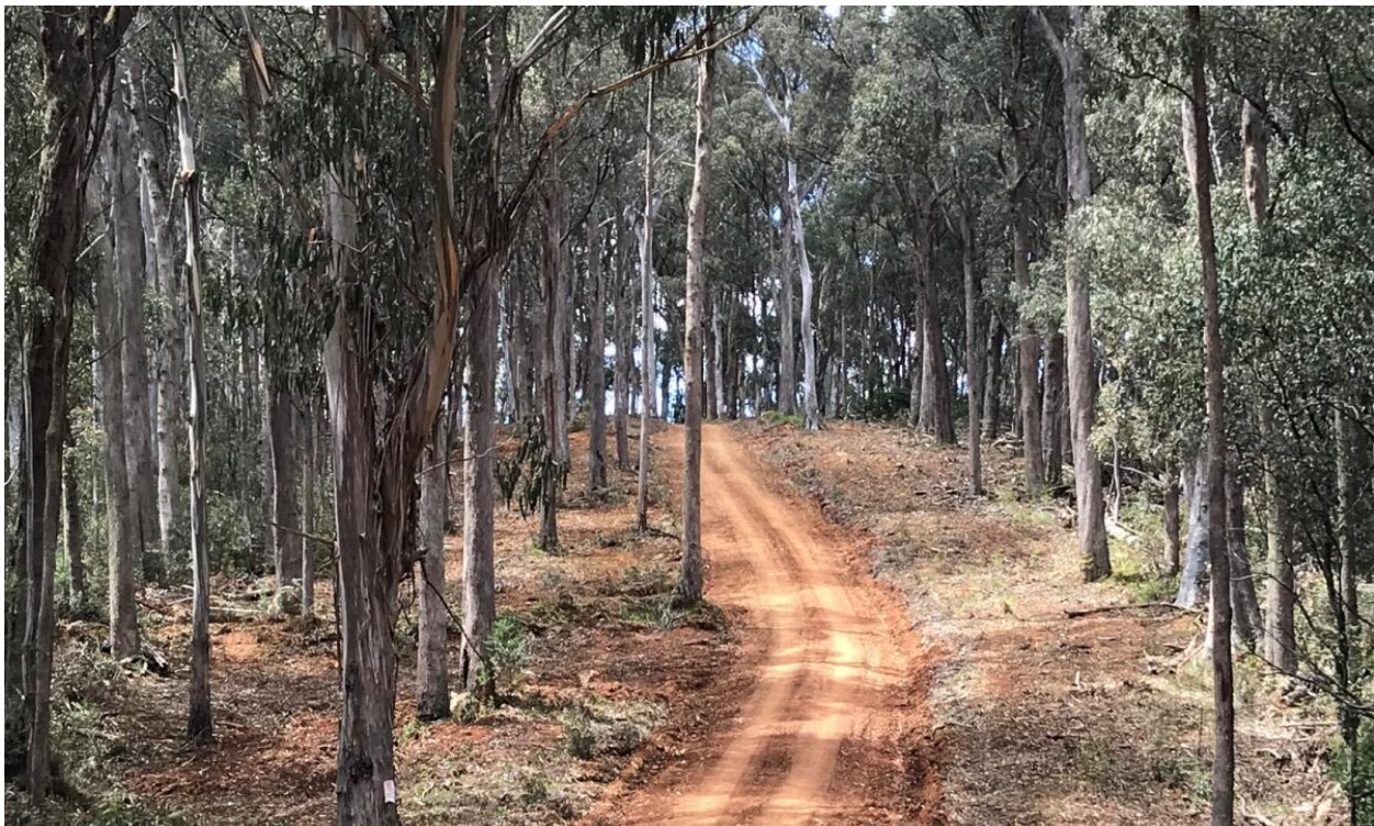
Figure 26. Forest clearing along evacuation route. Ladder fuels, undergrowth and small trees are removed for a wide corridor along the road. Crowns of trees along the road should not touch.
