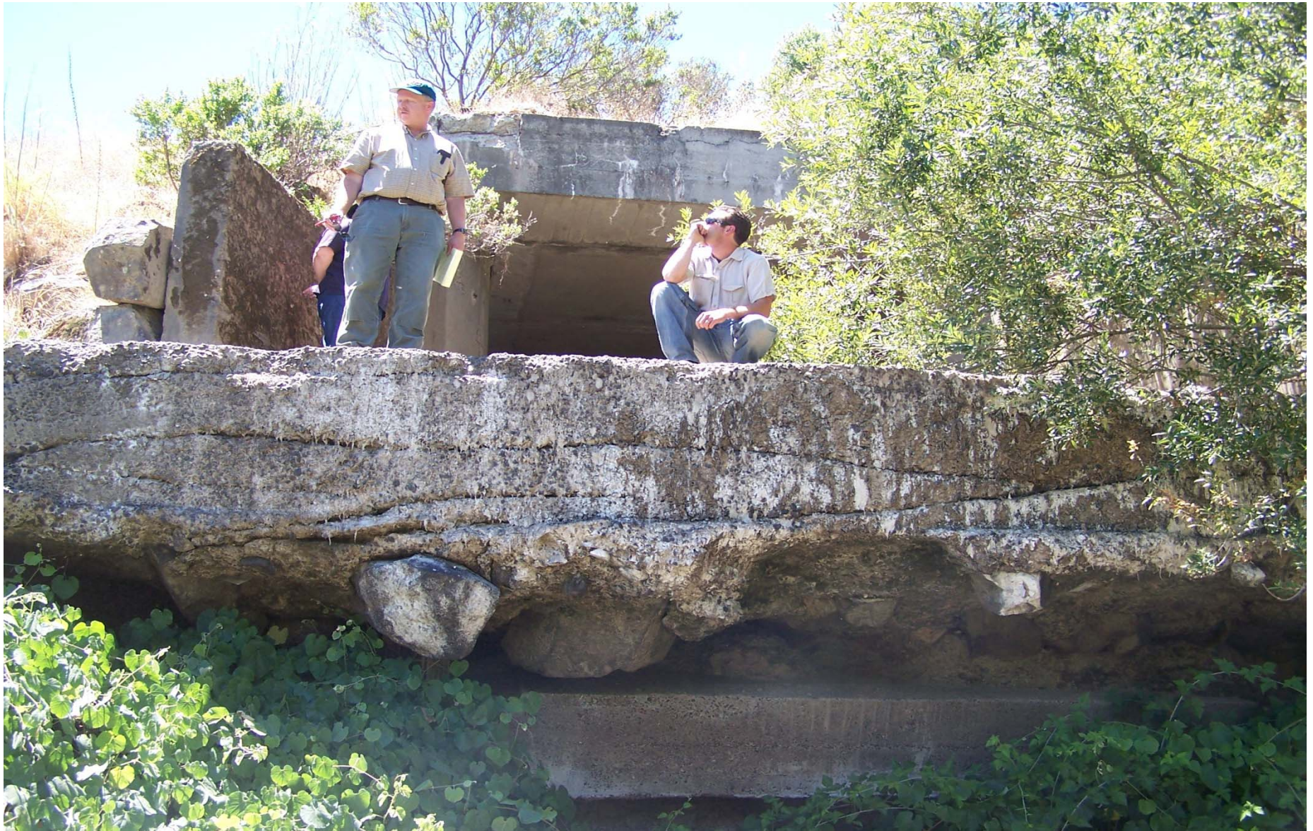
Box culvert of Storey Creek at confluence with Russian River hanging 20+ feet up on river bank and being under cut
