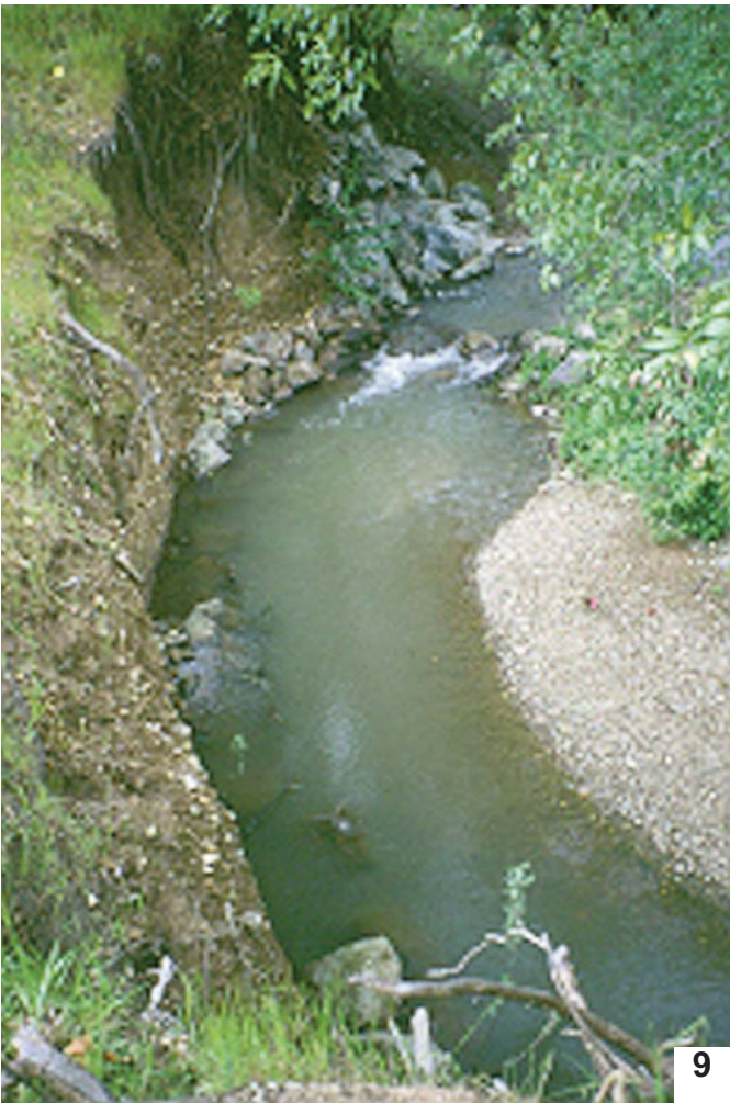
These photos show the undercutting and erosion around the willow walls indicating flow velocities continue to scour the channel due to the level of incision of the channel and the lack of a floodplain.
