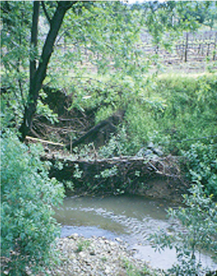
These photos show the undercutting and erosion around the willow walls indicating flow velocities continue to scour the channel due to the level of incision of the channel and the lack of a floodplain.
